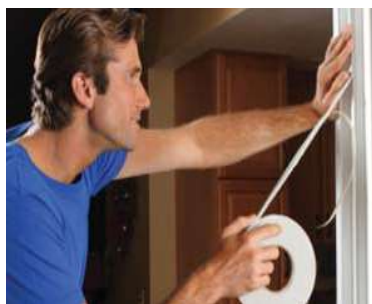
Fig 2. Installation of weatherstrips
